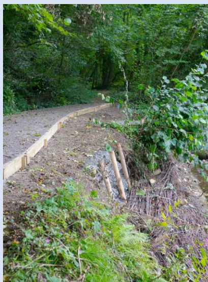
Image B: Reinstated path © BCBC
